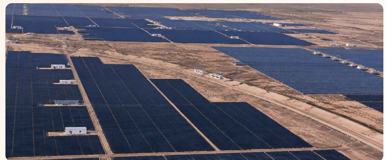
75 MW Group-Captive Solar Power Project
